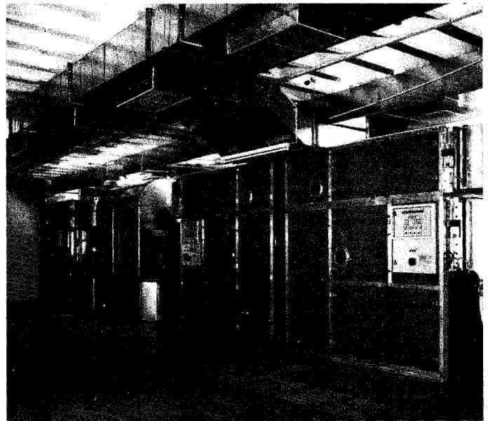
Ventilation and air conditioning units
